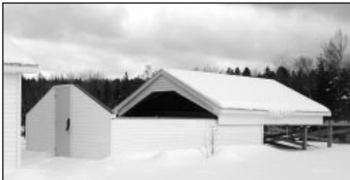
*The roll-off with the roof partially open.*
