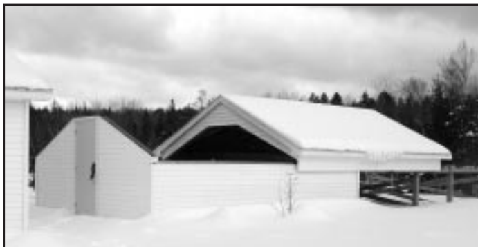
The roll-off with the roof partially open.
