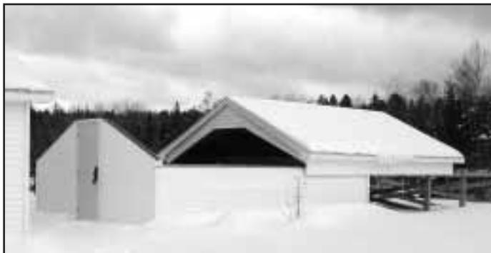
*The roll-off with the roof partially open.*
