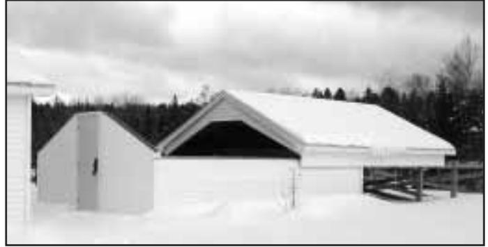
*The roll-off with the roof partially open.*
