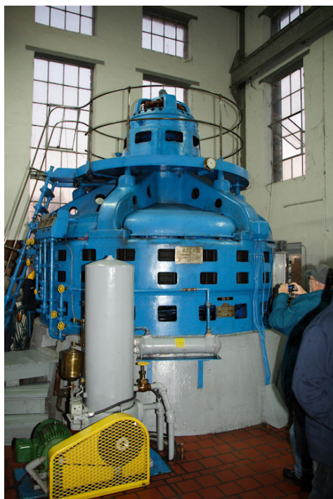
The lower 3 megawatt generator
