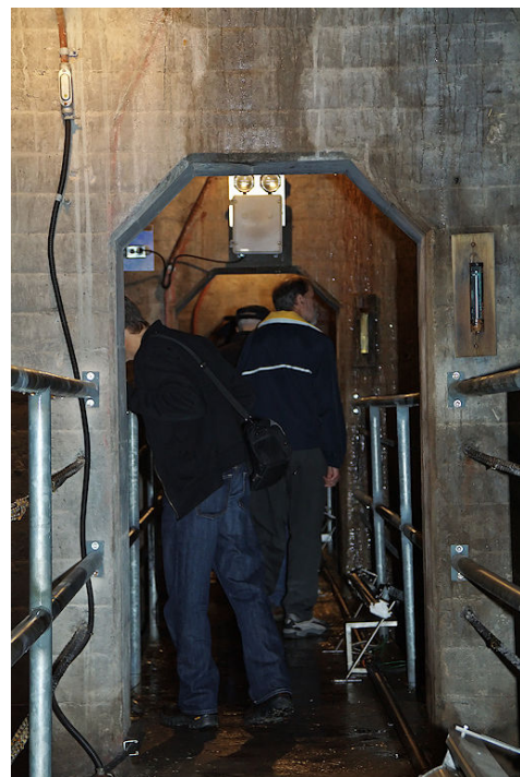
Inside the upper dam
