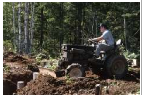
▲ Walter Urban of Avonport volunteered his time and tractor to back-fill the foundation columns for the roll-off track. (Sept 24th 1996)
