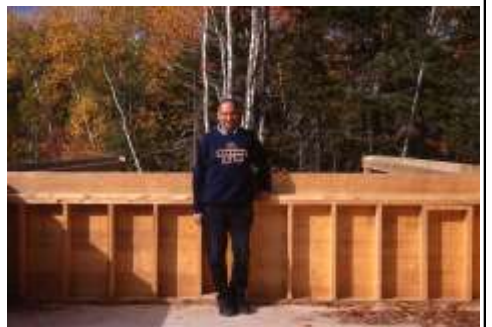
▲ David Levy (Nova East's 2012 special guest speaker) in the roll-off before the roof was constructed. (Oct 18th 1996)
