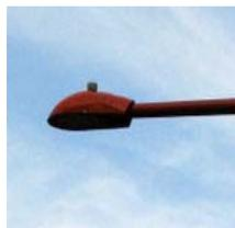
A flat-lens cobra luminaire, which is a full-cutoff fixture, may be effective in reducing light pollution. It ensures that light is only directed
