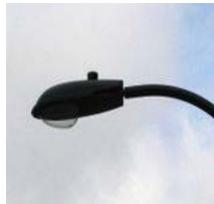
This drop-lens cobra luminaire allows light to escape sideways and upwards, where it may cause problems
